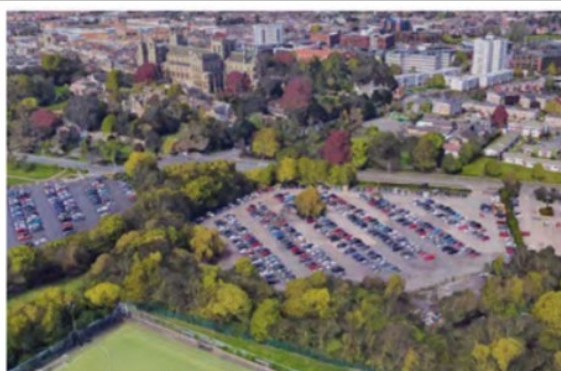
Aerial from south-east: Existing view
